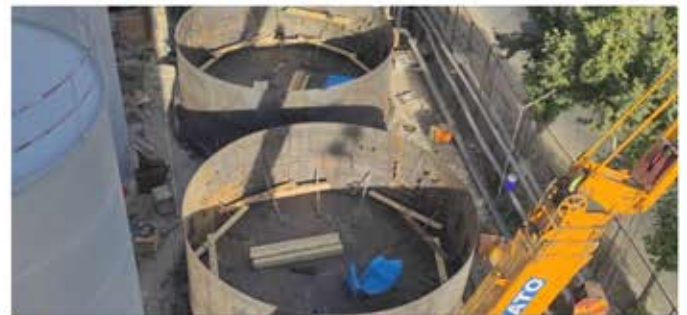
➤ Design and supply of materials and construction of 8 storage tank devices
