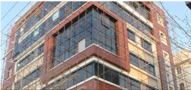
Six-storey residential and office building located in Vahid St., Tehran
