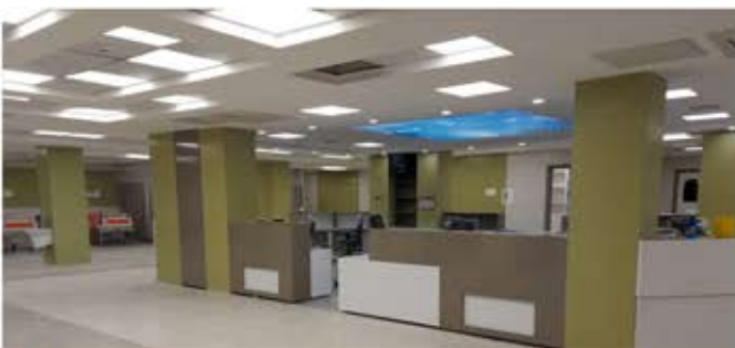
Repair and Reconstruction of the emergency department of Sabalan Hospital in Ardabil
