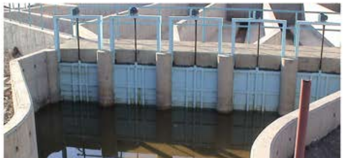
Qom drinking water treatment plant
