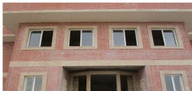
Birjand Wastewater Treatment Plant
