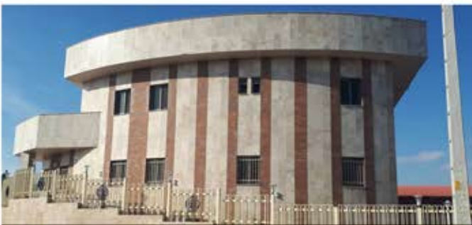
Construction and Installation of the Ajab Shir Social Security Clinic
