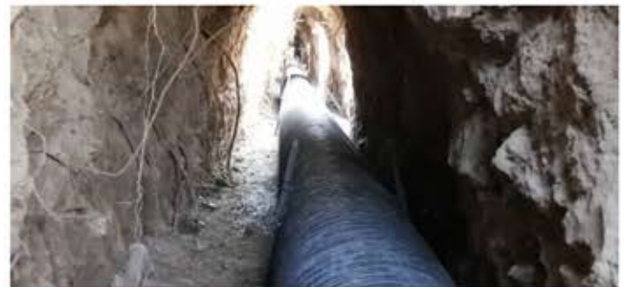
Design, construction and operation of wastewater collection and treatment systems in the zone 5
