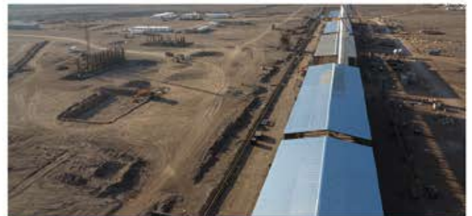
Construction and installation operations of Tabas Coke Factory
