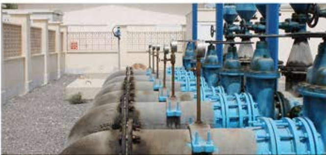
Construction of pumping and lifting stations for Kish Island sewage
