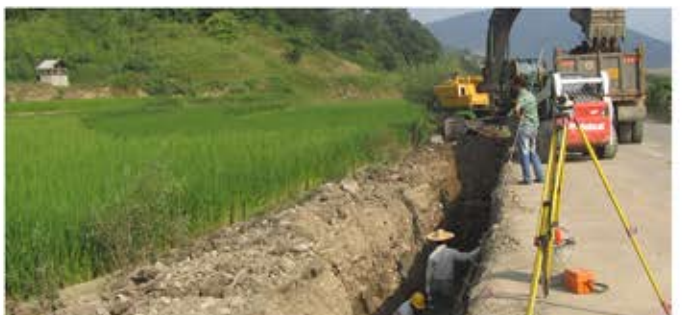
Construction and operation of Sari water transmission line and treatment plant
