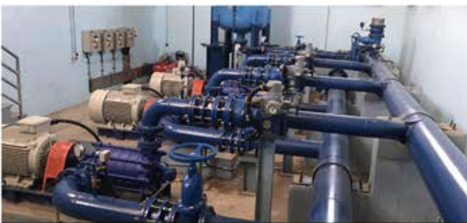
Execution of transmission line, access road and cathodic protection of Semnan water supply project from Roozieh fountain
