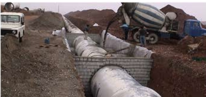
Qom drinking water treatment plant
