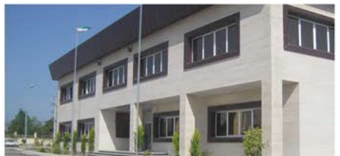
Construction and operation of the transmission line and treatment plant of the water transfer project to Sari
