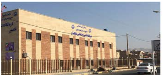
Construction and Installation operations of Delijan Social Security Clinic
